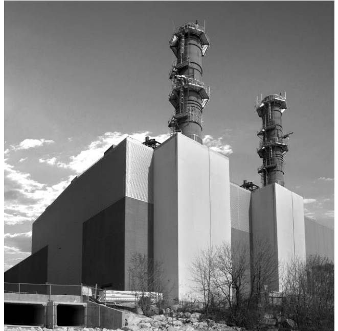
The first of two new natural-gas-fueled units at Port Washington Generating Station began commercial operation in July 2005.
